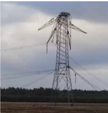
Storm damage caused by Hurricane Kyrill in 2007
