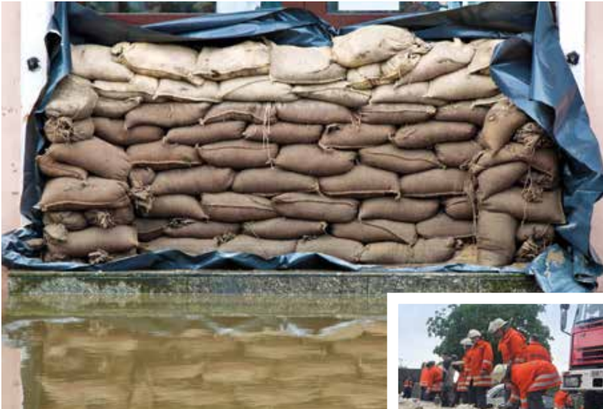
Protective walls of sandbags
